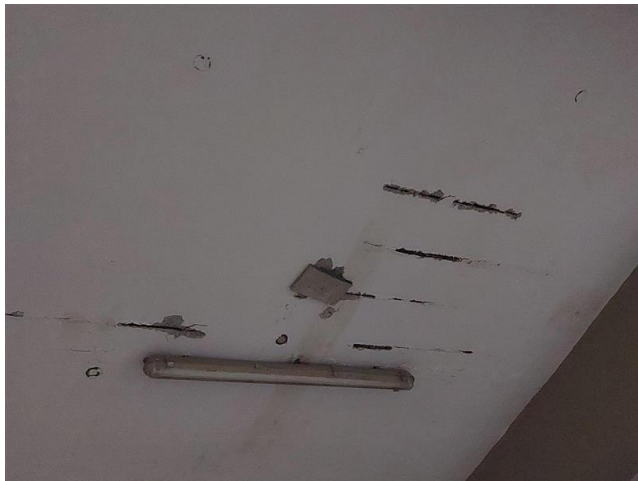
Figure 2: Exposed Reinforcement Bars under the Slab in Trench C.
